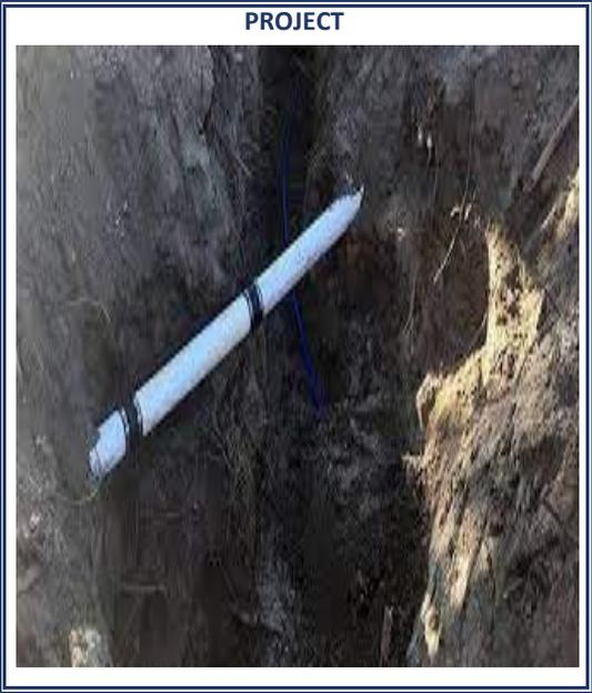
**PROJECT DESCRIPTION:** This project shall include the design & construction for the replacement of approximately 1,200 linear feet of undersized & deteriorating waterline in the Ehlers Road between Bluemont Scenic Drive & Tuttle Creek Boulevard. This project shall also include new 8-inch water main Spring Hill Lane, as well as a new water main extending from Bluemont Scenic Drive to Bluemont Circle. These two mains will be connected to the 24-inch main Bluemont Scenic Drive.
